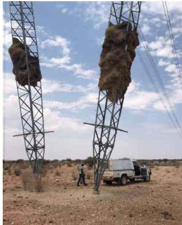
400 kV pole structures with birds' nests
